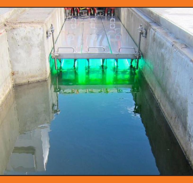
Horizontal Open Channel 6 PSI Ultraviolet Disinfection
